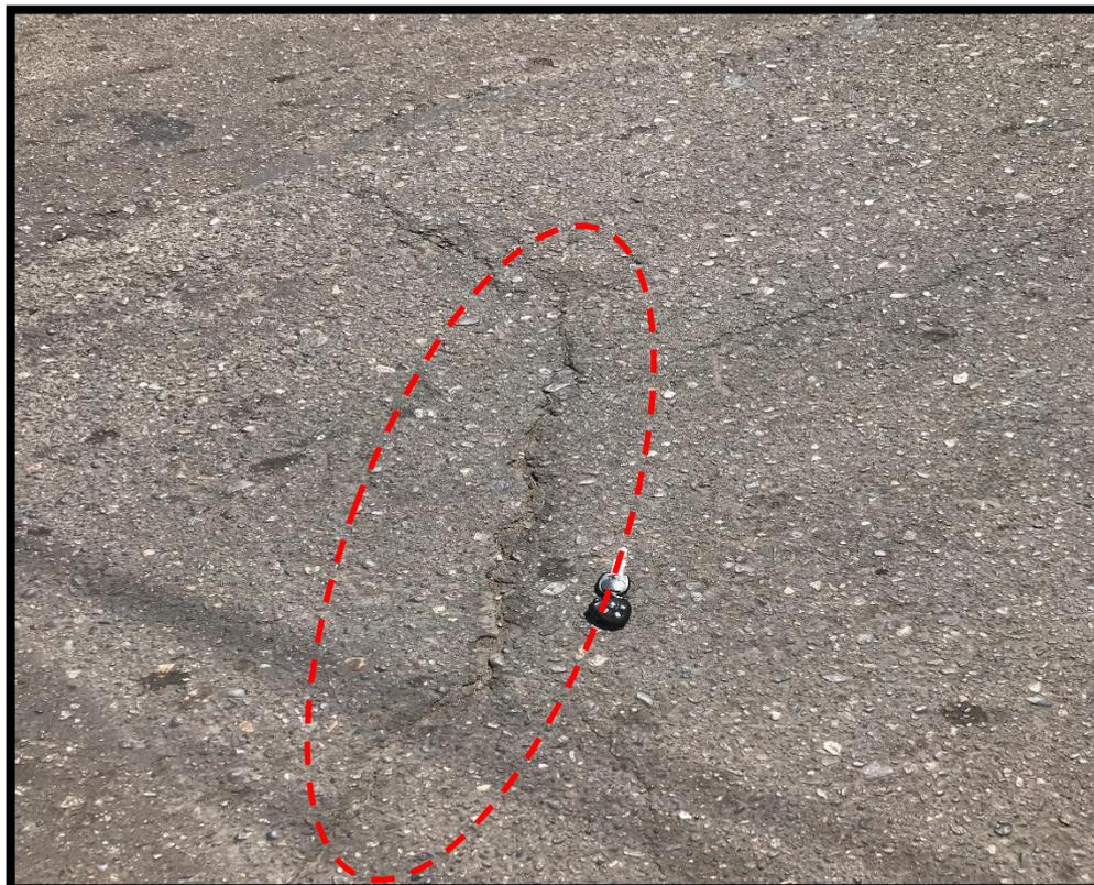
**FIGURA 3: AGRIETAMIENTO EN TRAMO ARIAS Y ARAGÜEZ**
