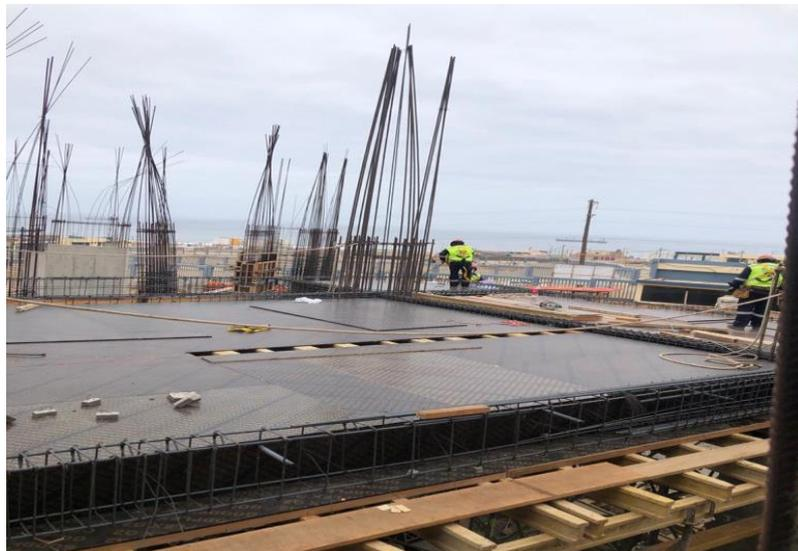
**Figura 8***Encofrado de Losas Macizas*
