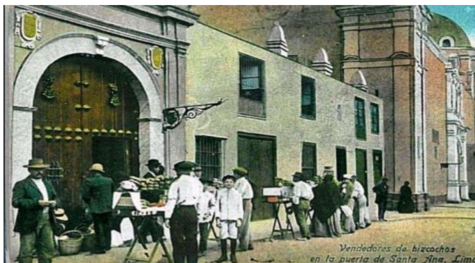
Figura 12: Hospital Santa Ana
