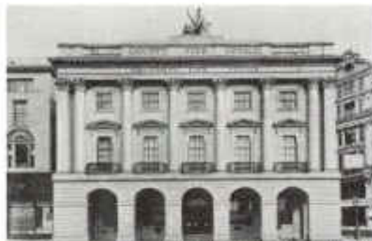
Figura 6 Country Fire Office
